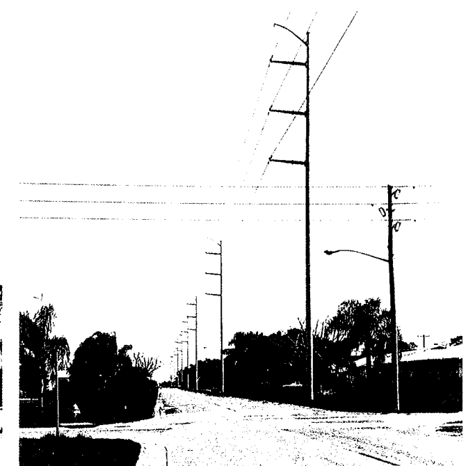
New single circuit 230 kv steel pole line on Lapp Horizontal Line Posts utilizes same narrow right of way through residential area. Clearances were maintained by putting all three phases on the street side of the pole.
