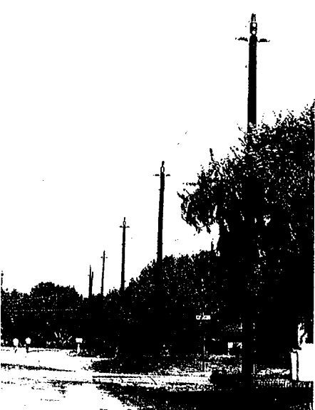
This trim looking, unshielded triangular configuration on wood poles combines economy and reliability in distribution construction.
