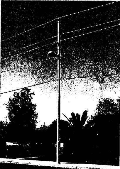
Unobtrusive distribution overhead in a residential area combines horizontal Distribution Posts and luminaire on same pole.
