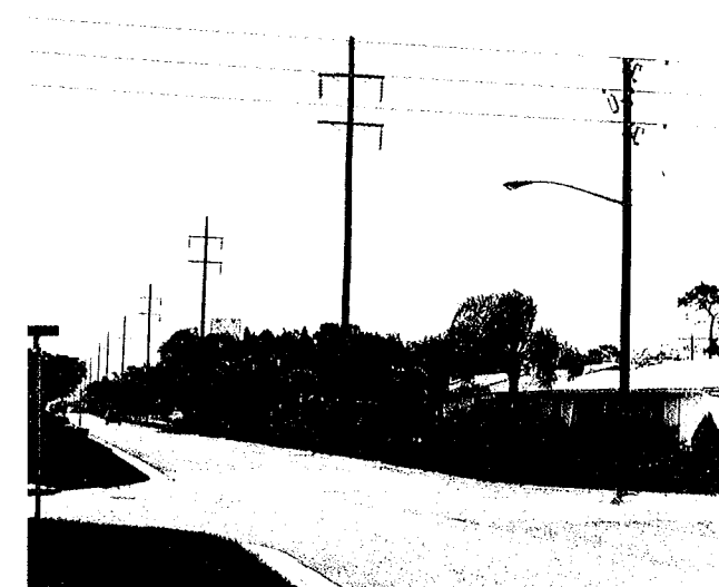
69 kv single circuit, tangent construction with suspensions on wood poles used only available right of way through residential area. Increased capacity was obtained by replacing and upgrading existing line to 230 kv. (See photo to the right).
